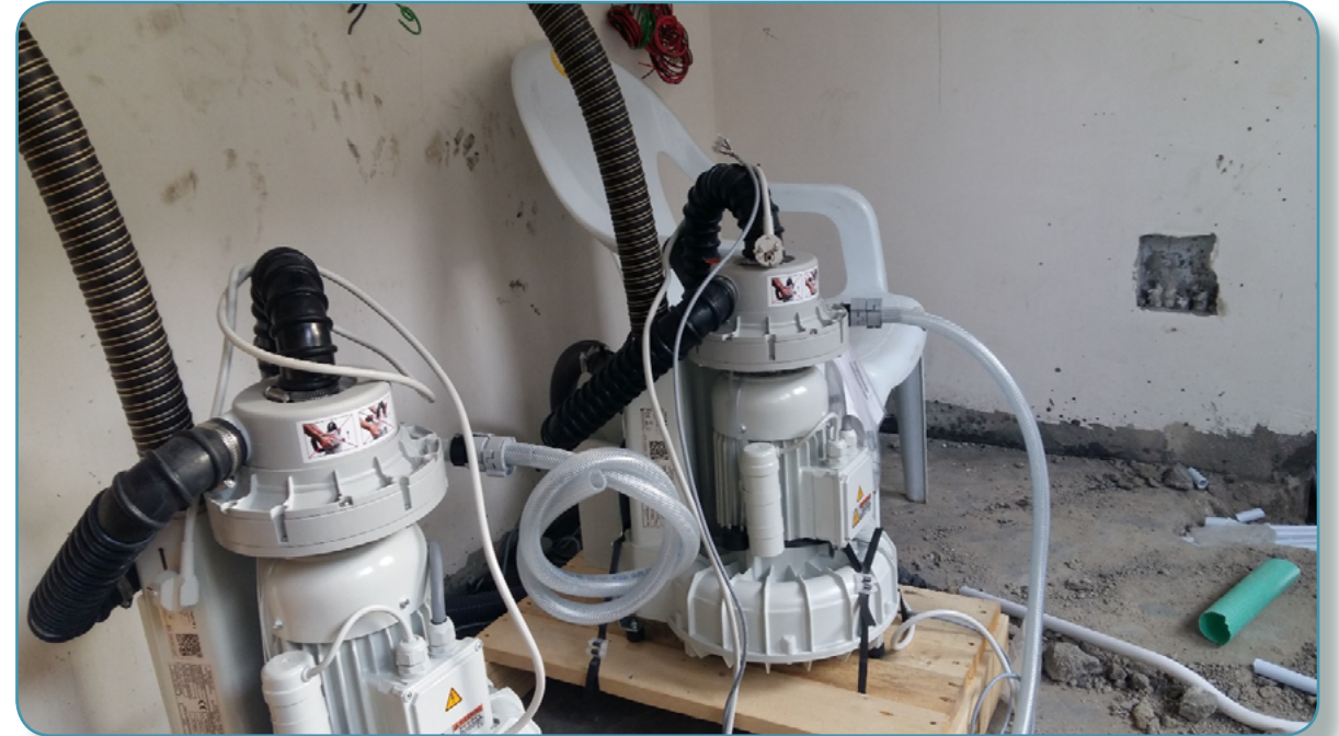
Mechanical room : Installation of compressors and suction pumps
