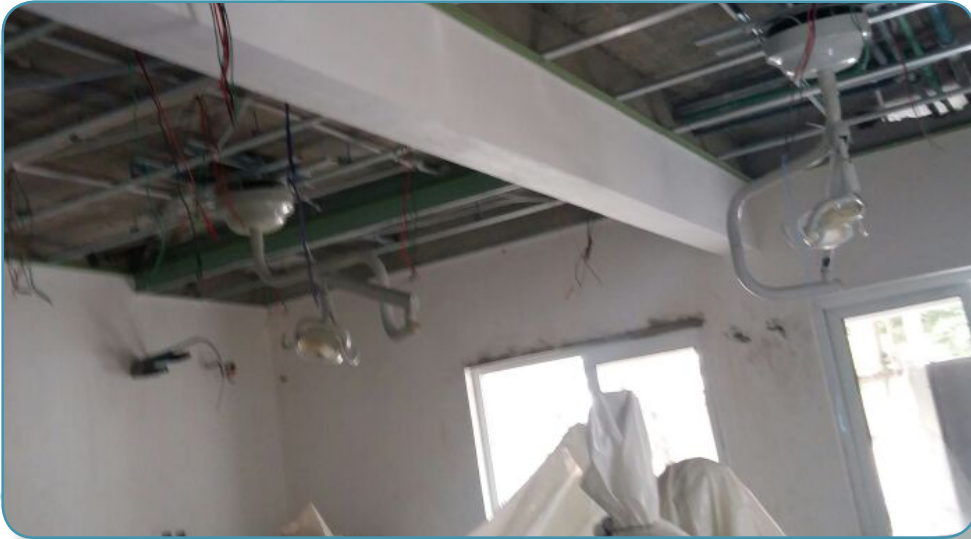
Installation of ceiling lamps
