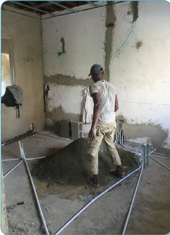
Pre-installation - Installation of pipes and electric wires
