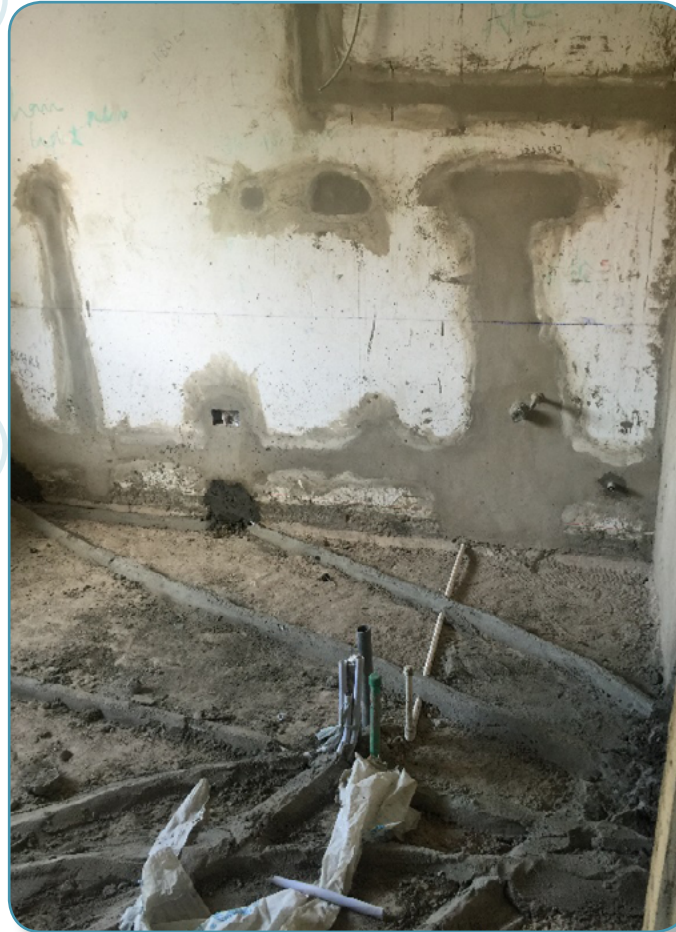
Pre-installation - Installation of pipes and electric wires
