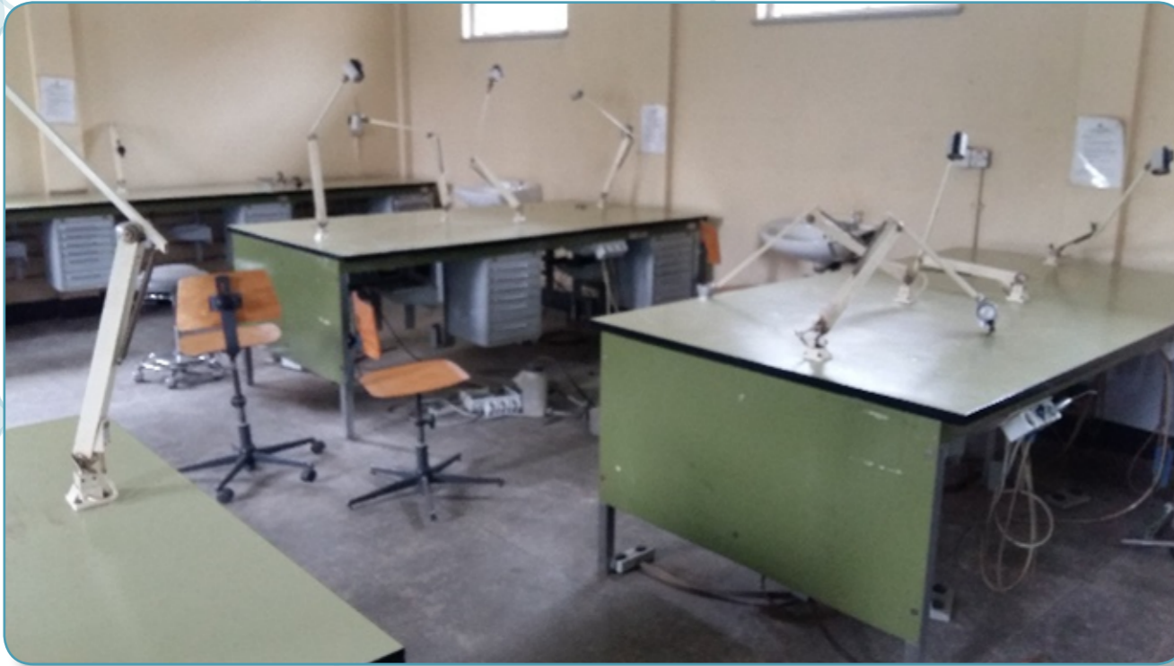
Practical work room before refurbishment
